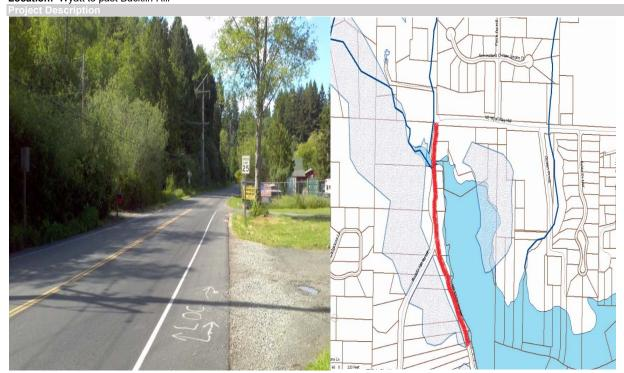
Description: Current level of service E for Pedestrians and D for cyclists. Provides shoulder widening on both sides. Necessitates upgrading Cooper Creek Culvert to accommodate road widening. Involves ROW acquisition. Assumes additional land will be needed to mitigate displaced wetlands. Desirable to improve curb radius at bottom of Wyatt.
